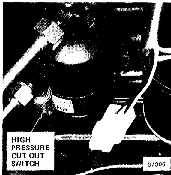
Figure 4 - RH Front Engine Compartment
